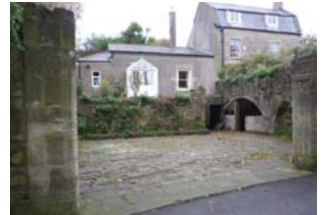
The locally important buildings make a significant and positive contribution to the character of the Conservation Area
