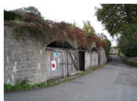
The brewery vaults of the former South Stoke Brewery
